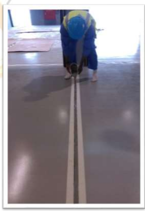
Joint Sealant Application
