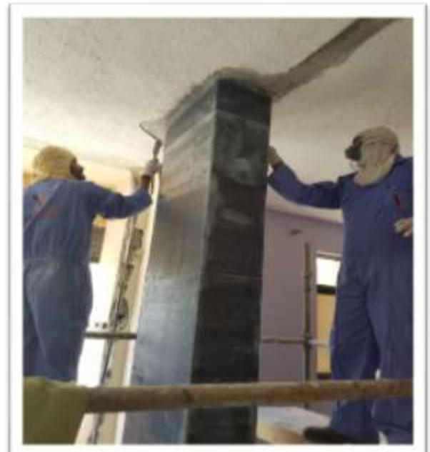
Carbon fibre wrapping 1 st layer, after completion
