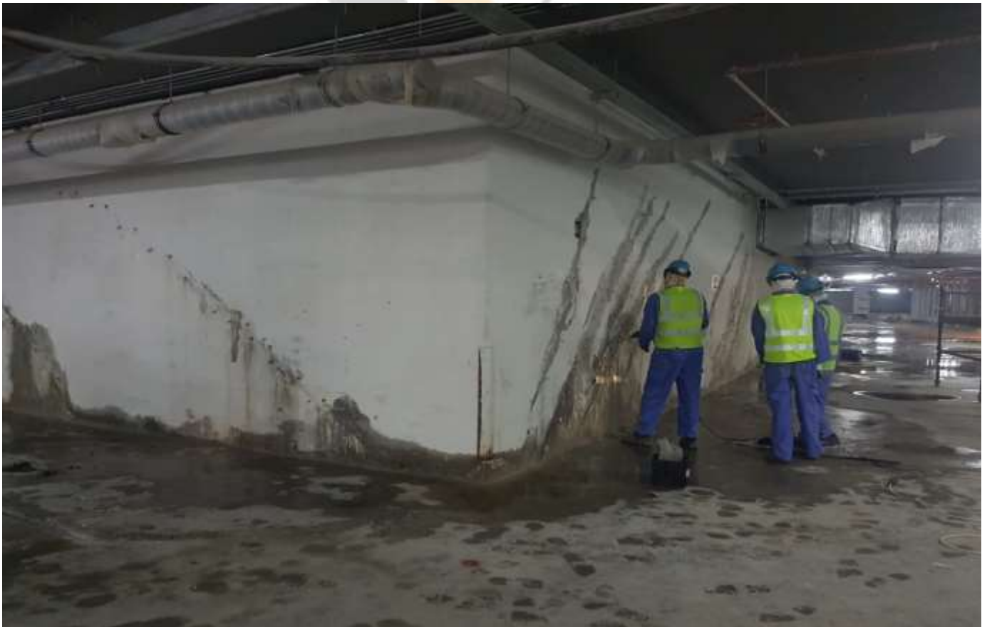
Polyurethane Leakage Injection Works
