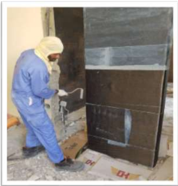
Carbon fibre wrapping 1 st layer, after completion
