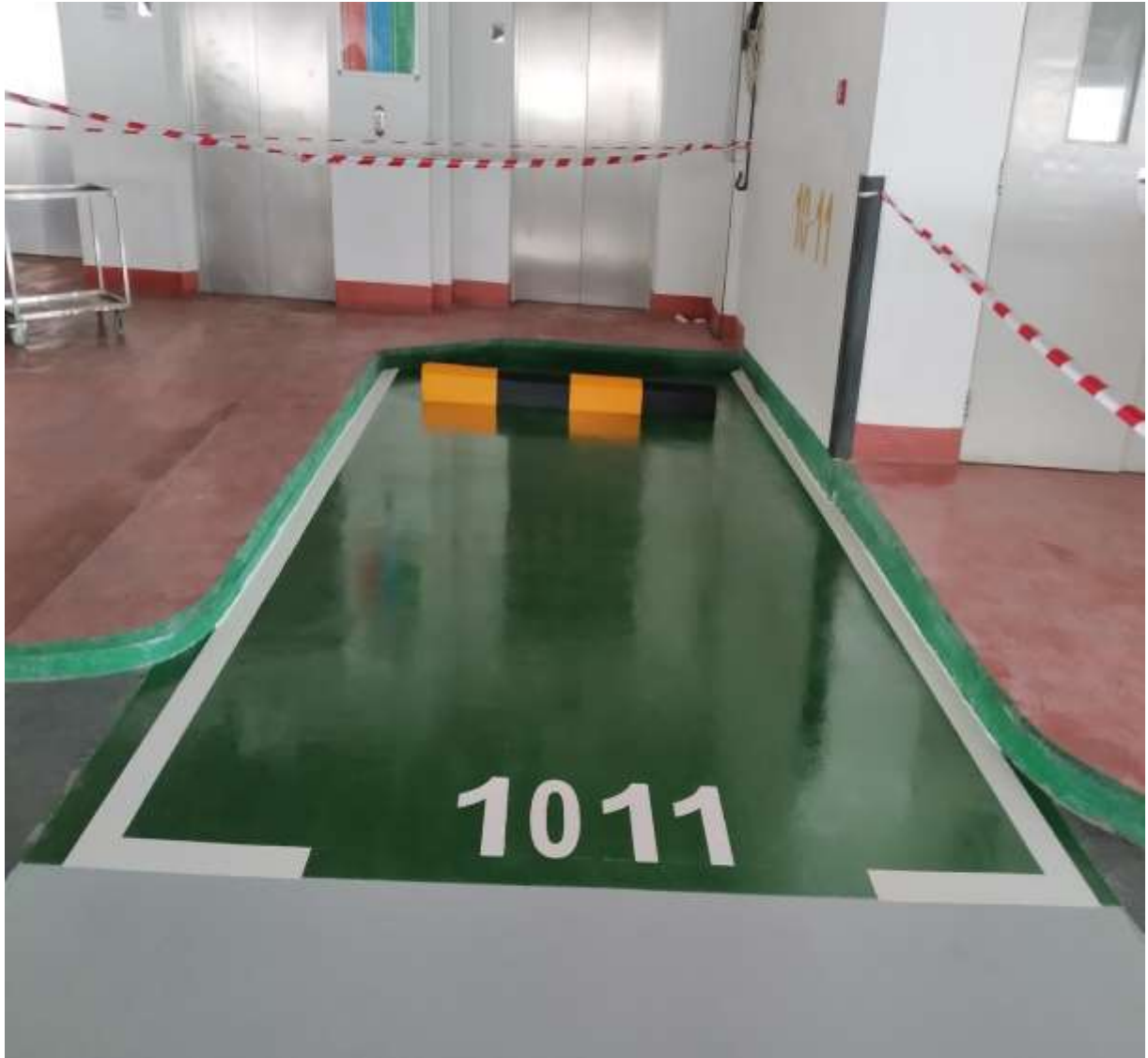
Car Park coating works at Al Zahra Hospital
