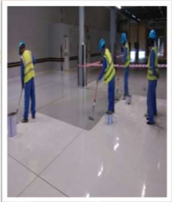
Top Coat Application
