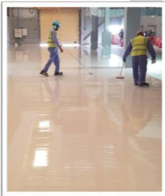
Base coat levelling by Spike Roller
