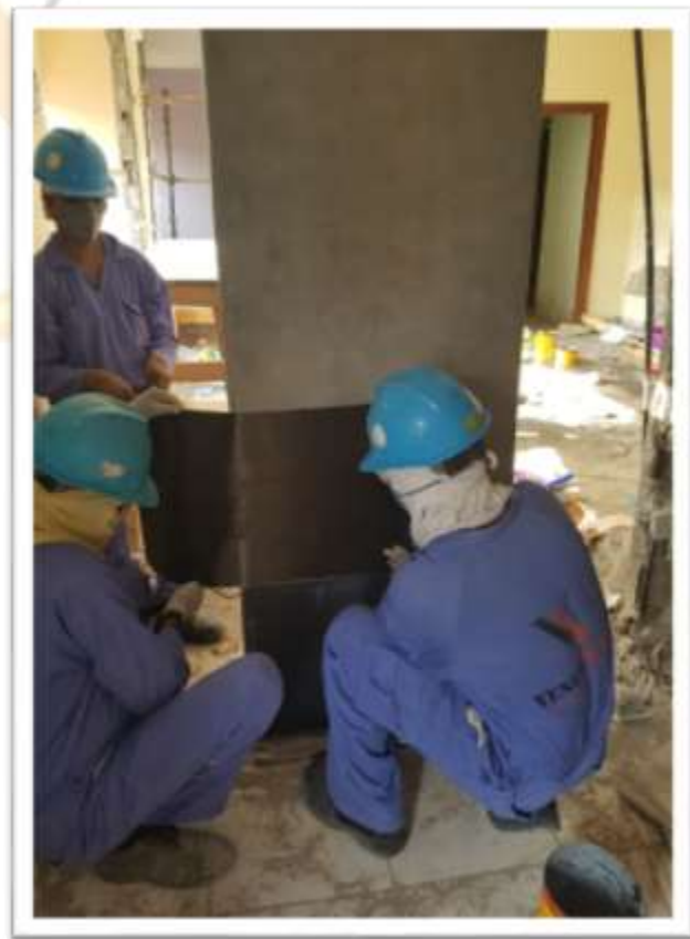
1 st layer of Carbon Fibre Wrapping to the Column
