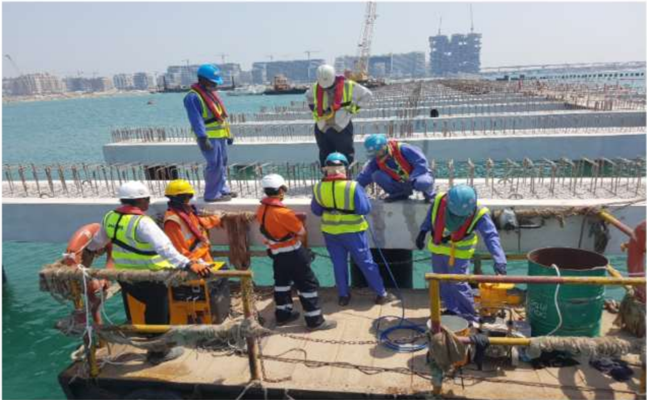
Dry Crack Injection works In Dubai Harbour
