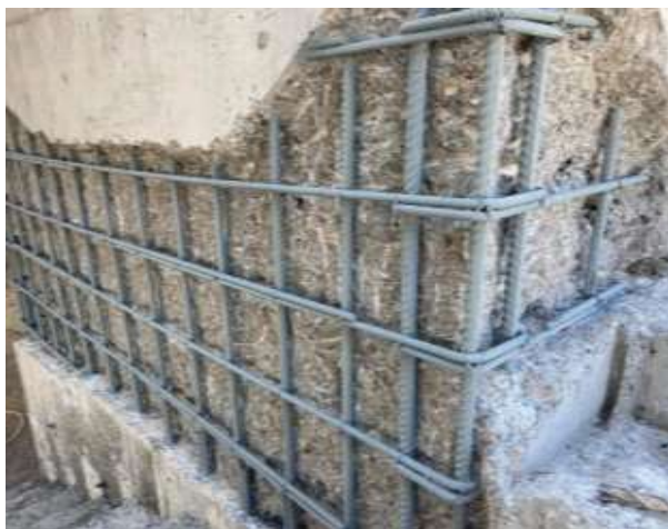
Concrete Repair Before Work:
