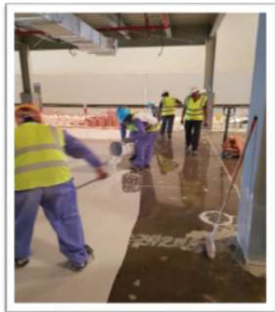
Base Coat Application
