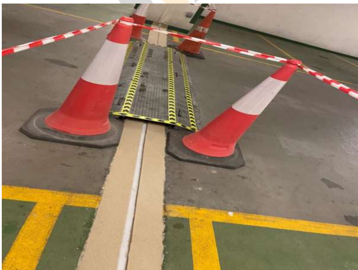
Expansion Joint Repair works in Abu Dhabi Mall
