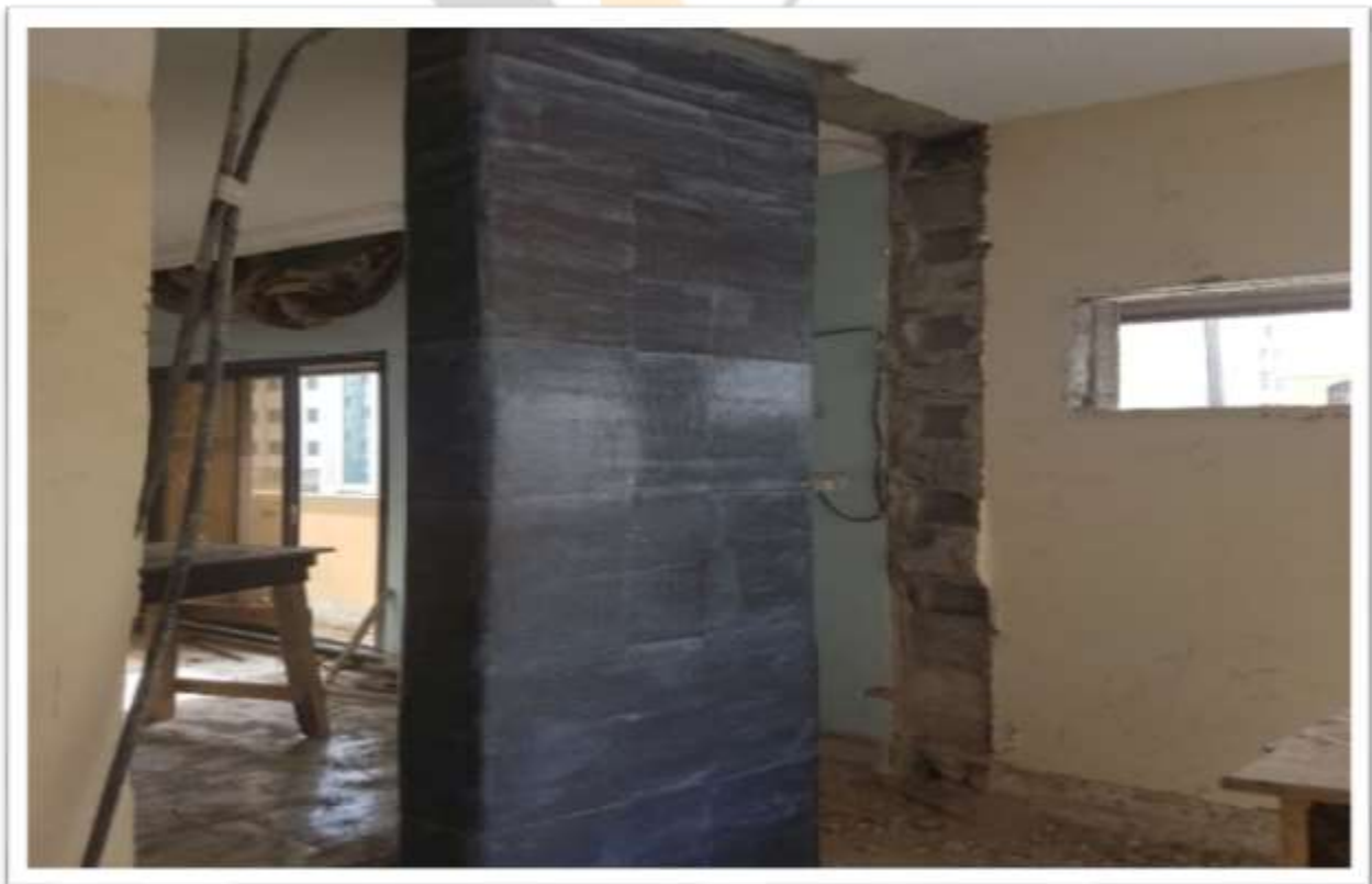
2 nd layer Carbon fibre wrapping
