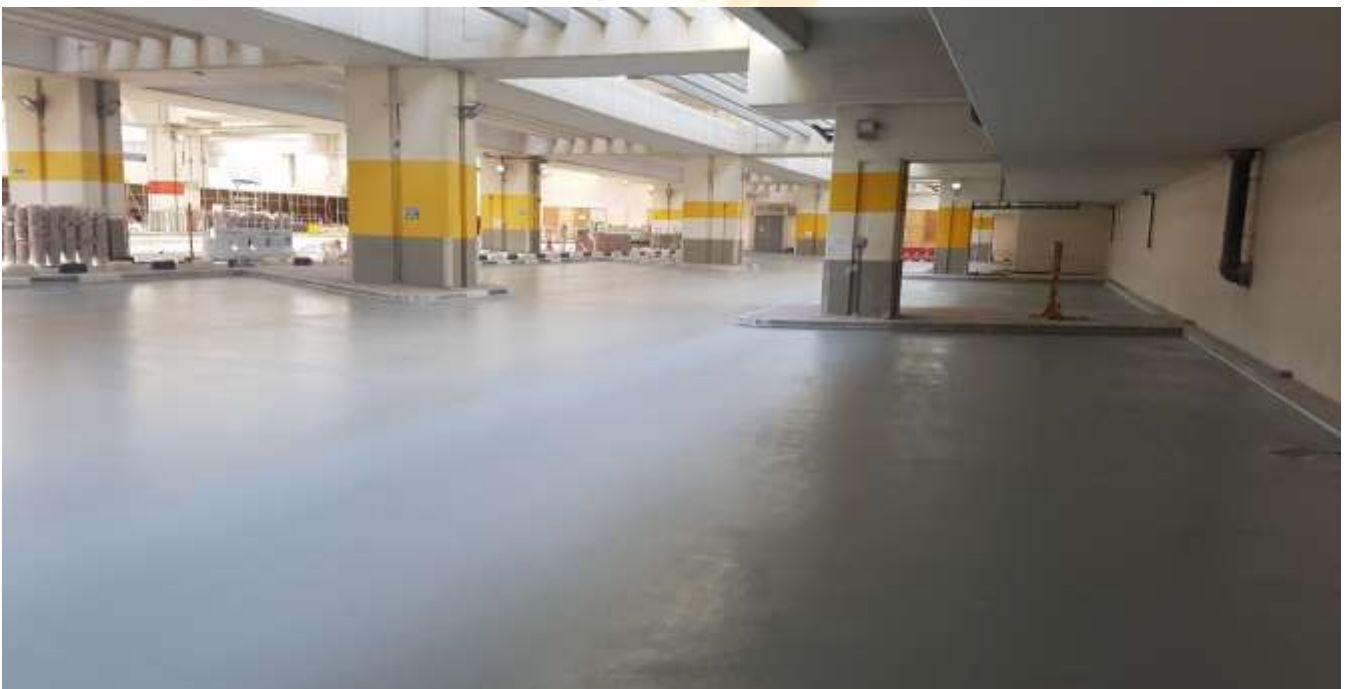
Polyurethane Floor coating works at Dubai Airports-Terminal 3 (Arrival Parking Area)
