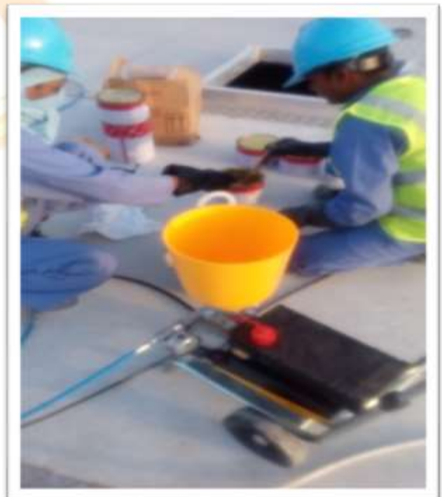
Polyurethane Leakage Injection
