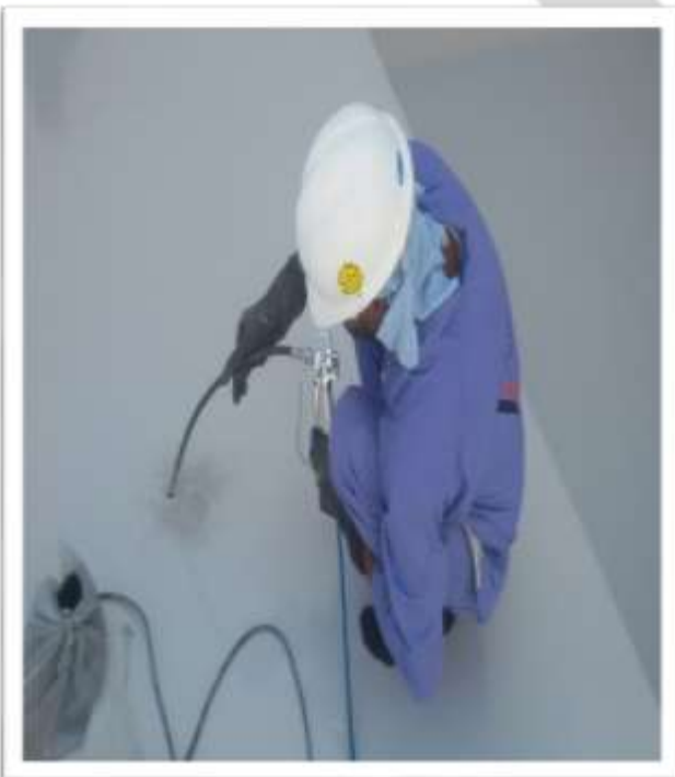
Polyurethane Leakage Injection
