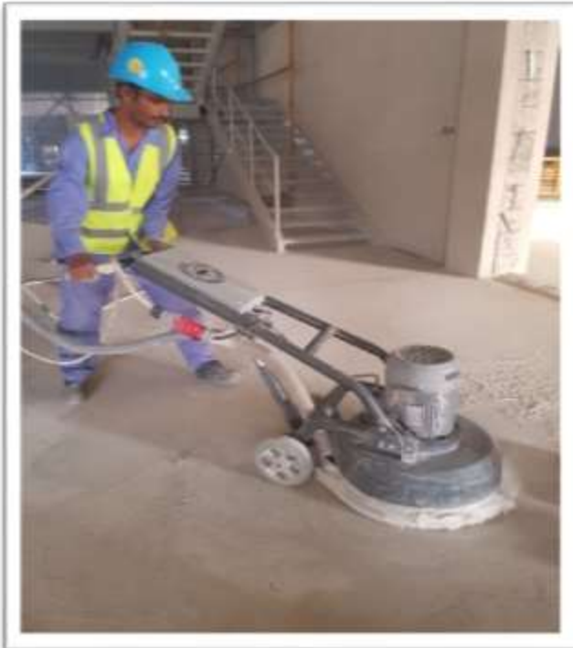
Floor Grinding
