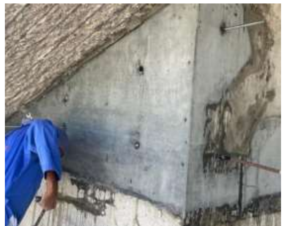
Concrete Repair after work
