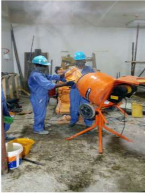
Micro Concrete Mixing
