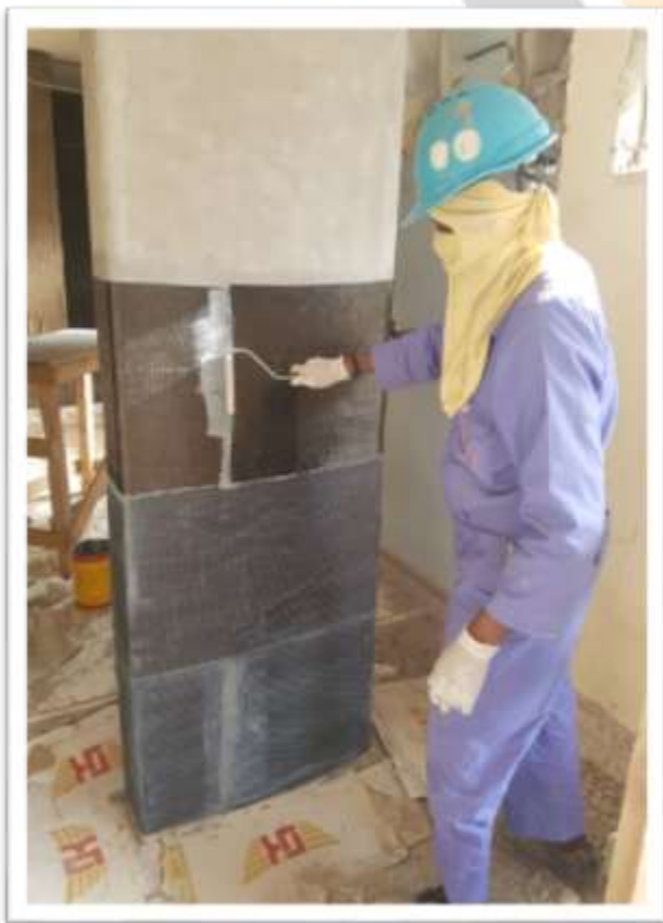
1 st layer of Carbon Fibre Wrapping to the Column
